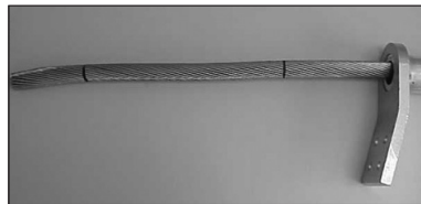
FIGURE 3: Slide aluminum dead end body over conductor.
