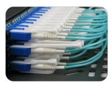
LC uniboot patch leads allow maximum access to the patching environment.
