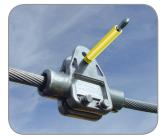
5. Remove the "Hot Stick" from the Live-line Attachment Tool
