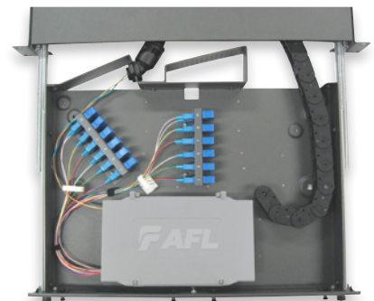
Fusion splicing of loose tube cable (24 fibres)
