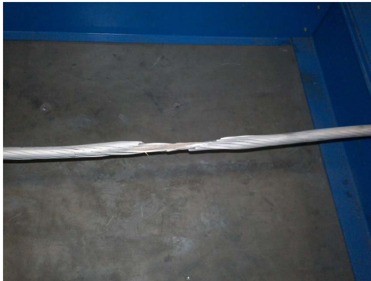
Figure 2 - Sample 2 full conductor break location
