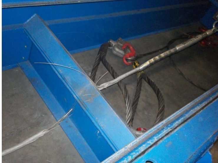
Figure 3 - Sample #2 full conductor break location
