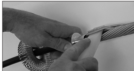
FIGURE 7: Pry Structural Reinforcing Rods over Split Corona Sleeves.
