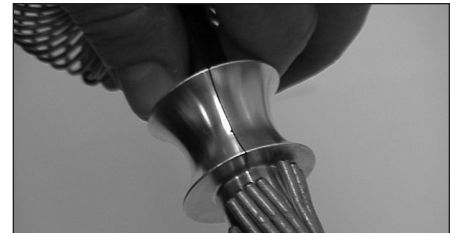
FIGURE 8: Align ends of Structural Reinforcing Rods over Split Corona Sleeves.
