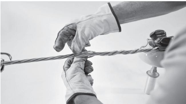
7. One side is now complete. Repeat steps 3-6 to the other side with the second tie. (Note: Wrap the tie over the pad in this installation.)
